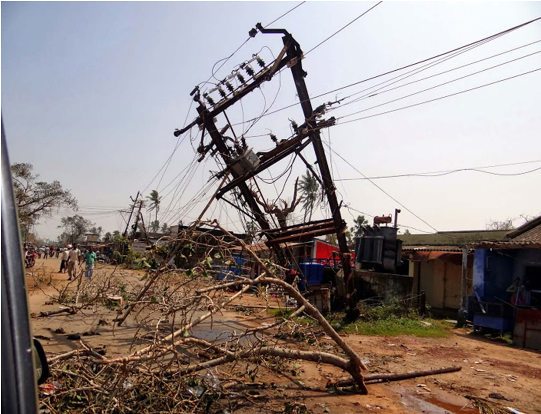
As greenhouse gas emissions continue to rise and climate impacts worsen, dramatic loss of life, assets, income and territory are becoming all too common. Here, damaged trees and electricity pylons lie strewn across a road after cyclone Phailin struck eastern India in October 2013. (Credit: © CARE).
