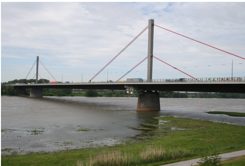
A1 Leverkusen bridge - Source: Pro Mobilitaet
