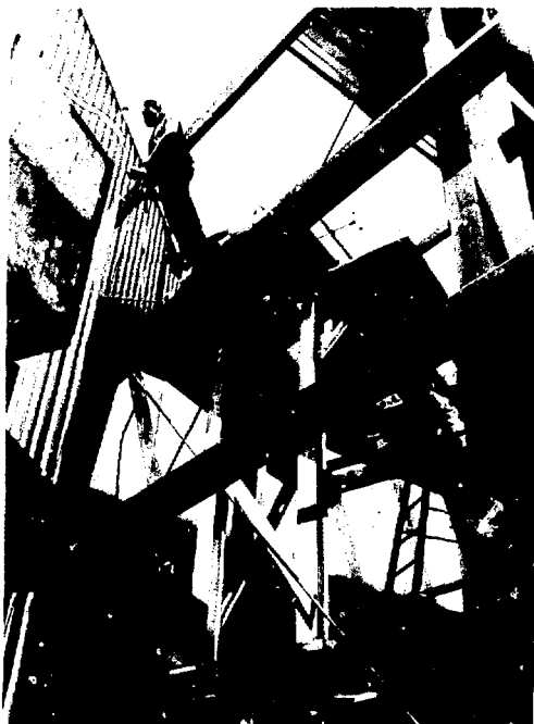
Figure 6. Experiment 755 (BNL/Minn/SE Mass) under construction.
