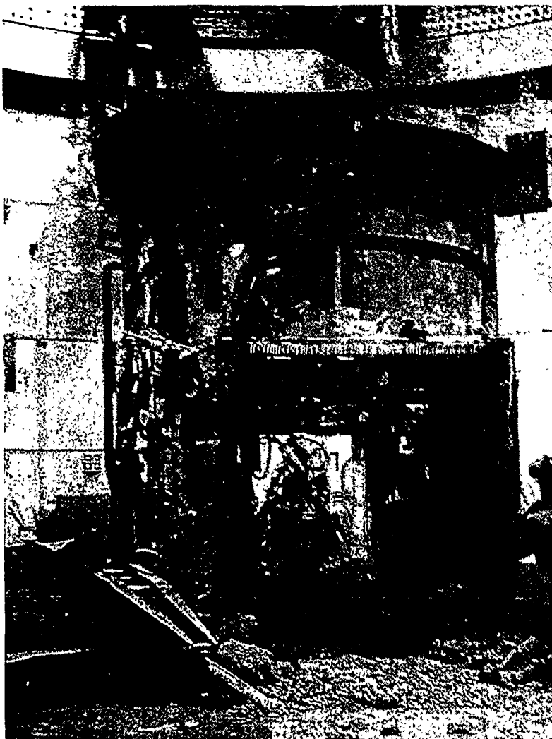
Figure 1. CP-5 reactor tank with bioshield and lead removed.
