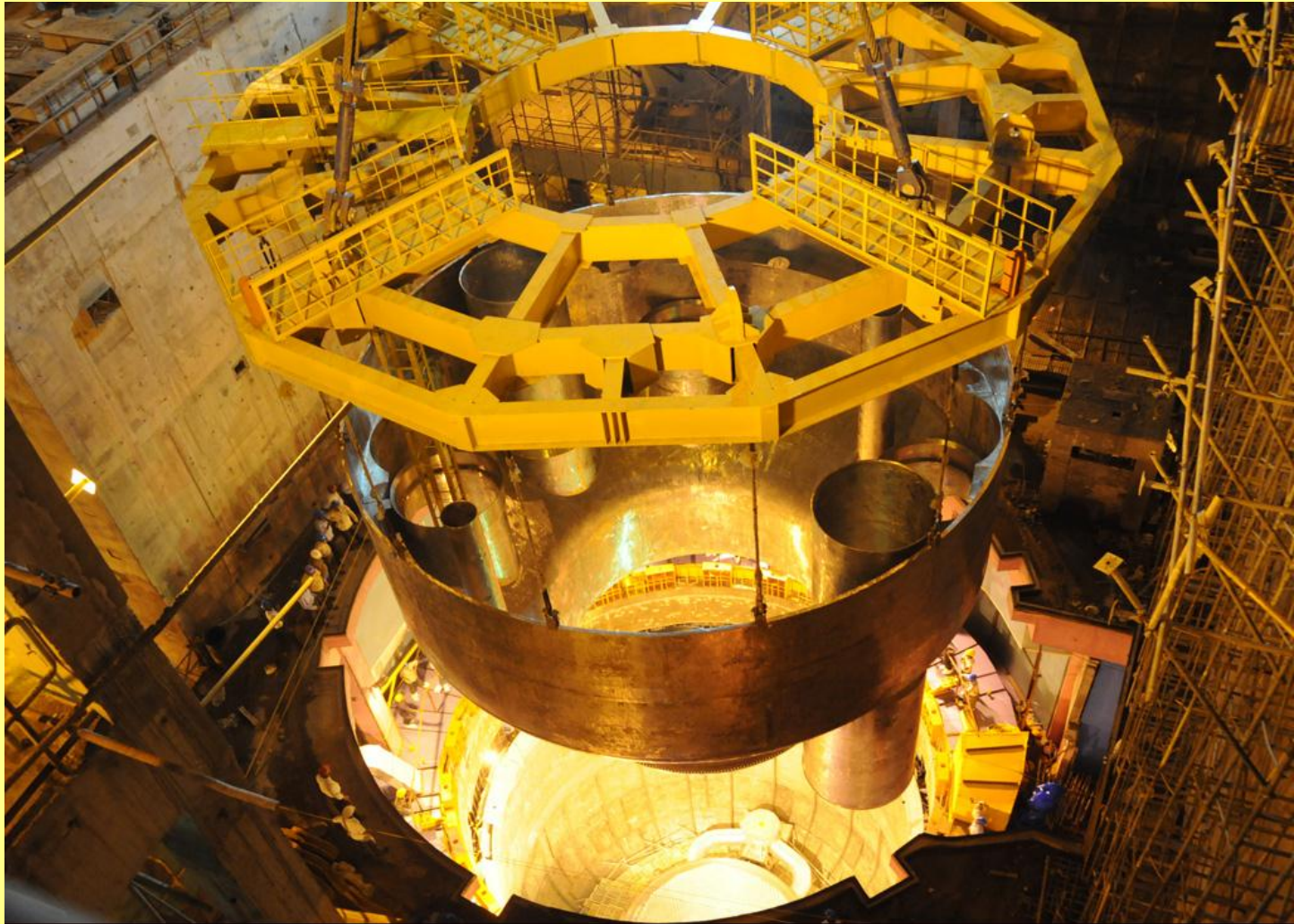
Inner vessel erection
