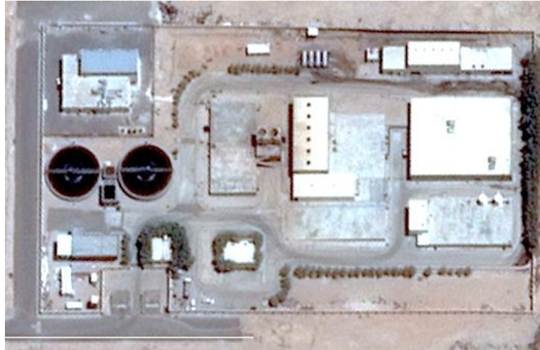
Figure 1 Aerial view of HBT desalination plant
