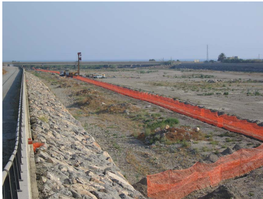
FIGURE 2. Excavation of the ALERT trench and drilling
