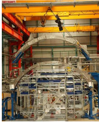
Figure 5 : OIS installation onto a TF coil
