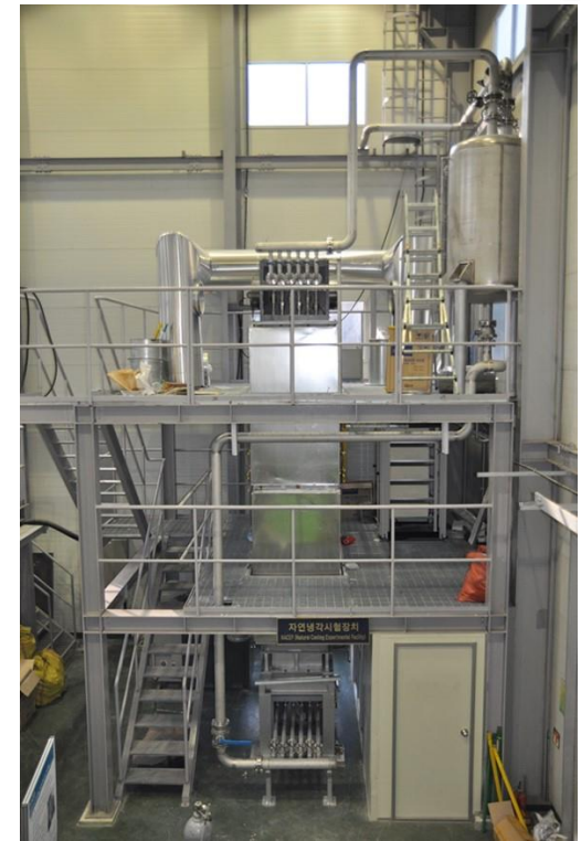
KAERI Hybrid RCCS Test Facility
