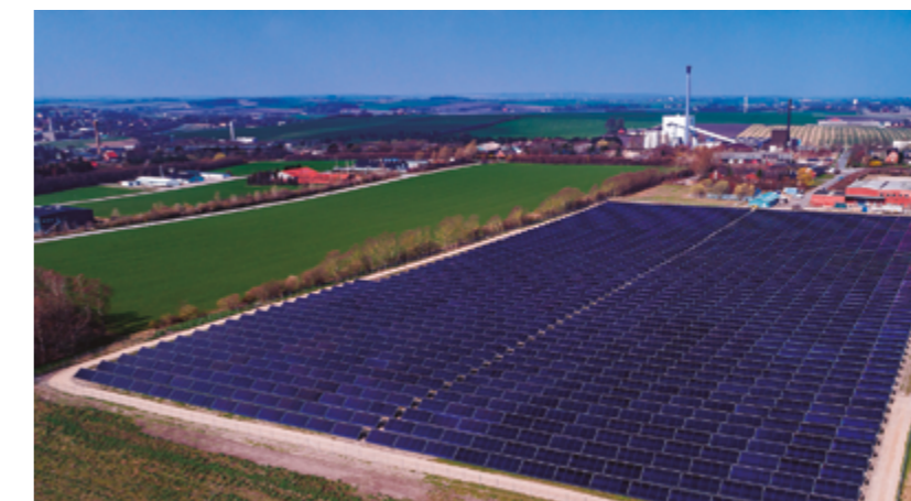
14.5 MW collector field intalled on a former industrial site PHOTO: SAVOSOLAR
