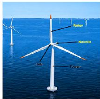
Figure 4: Hybrid wind turbine system [62]
