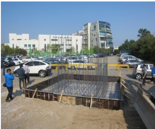
Figure 10. Arrangement of reinforcement and installation of foundation forms.
