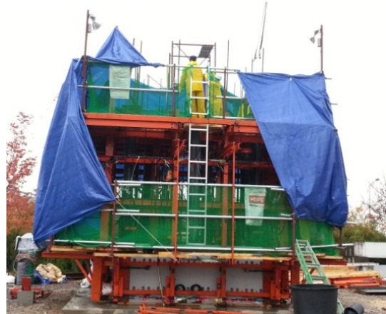
Figure 13. Installed slip form system.
