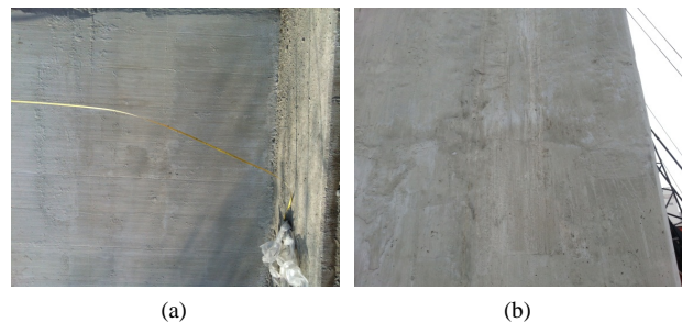
Figure 15. Surface of concrete. (a) Surface wave velocity < 1100 m/s; (b) Surface wave velocity > 1100 m/s.
