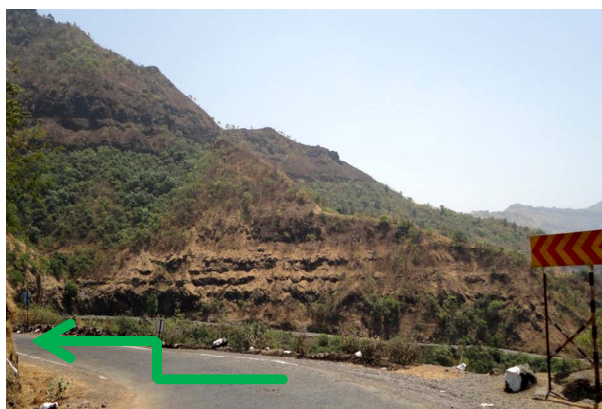
Figure 1. The panoramic view of the hill slope.
