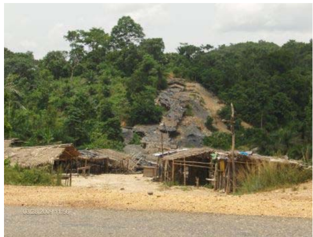
Figure 3. Shallow underground workings at right angles to road and likely to have traversed it.
