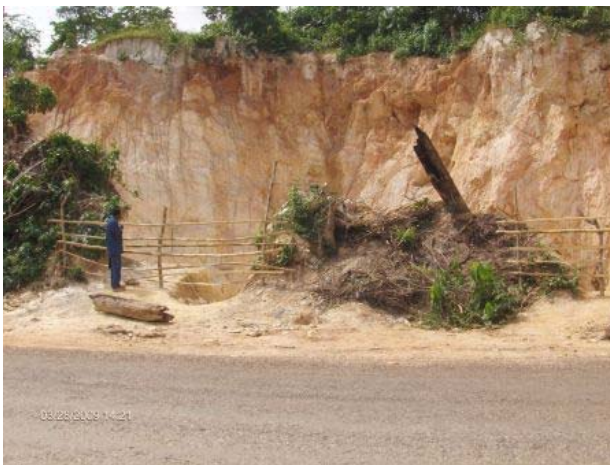
Figure 5. A 20 m deep pit worked on the cut slope of the road at Nsoupon near Dadieso.
