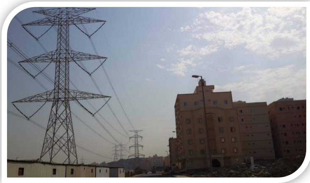
Figure 8. Proximity of high-voltage towers to nearby buildings.
