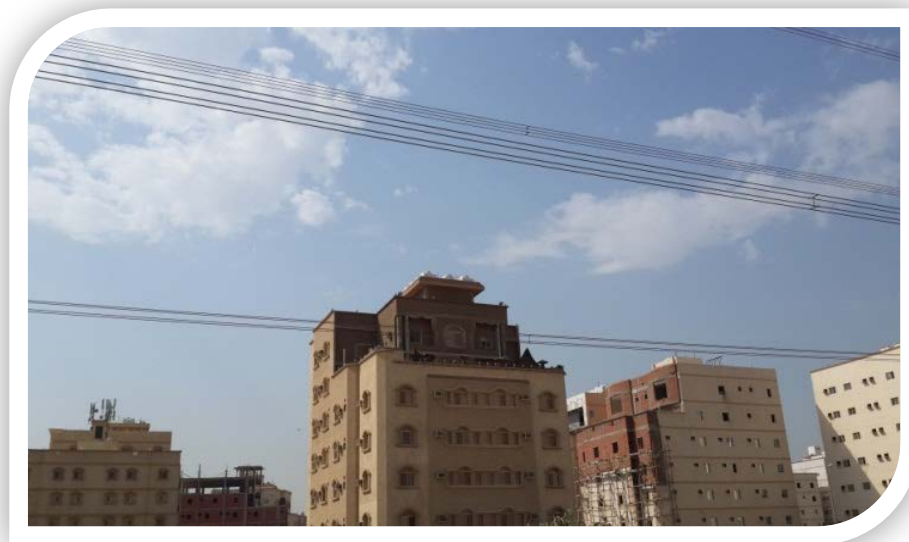
Figure 7. Proximity of power lines.
