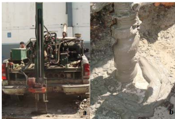
Figure 1. (a) Hydraulic punch employed at the sampling process; (b) Helicoidal drilling device.
