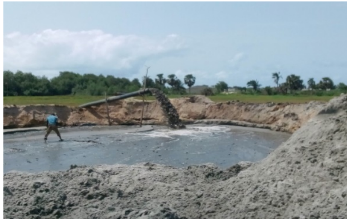
Figure 6. Sand dredging at the Ganganzoumè site.
