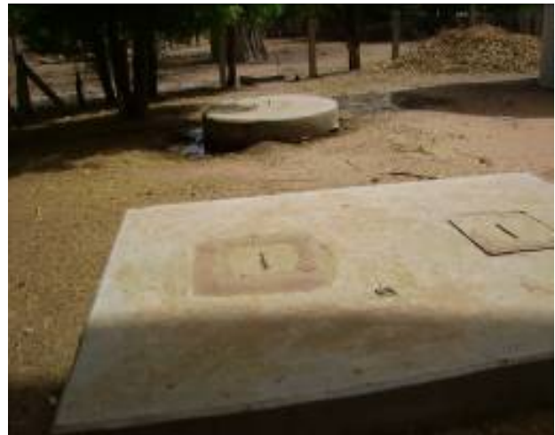
Figure 7. Tank and soakaway e.
