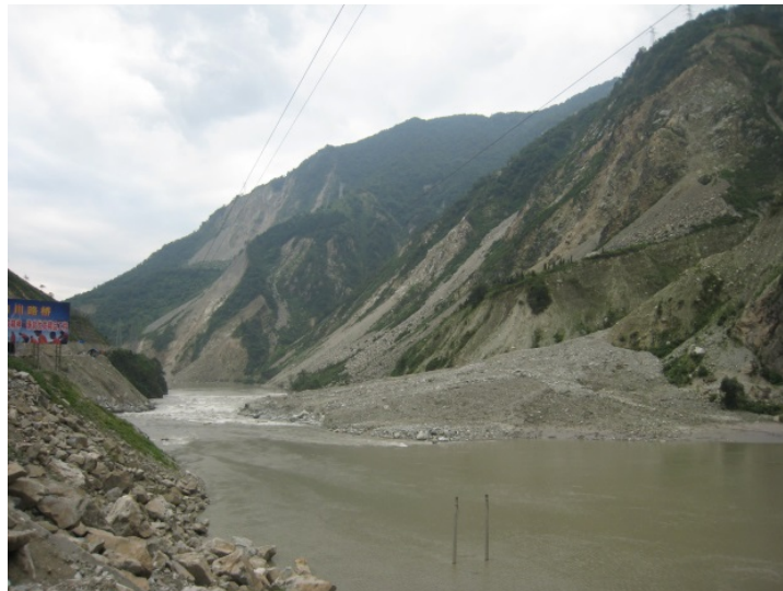
Figure 2. Dammed lakes formed by gully debris flow at Min River.
