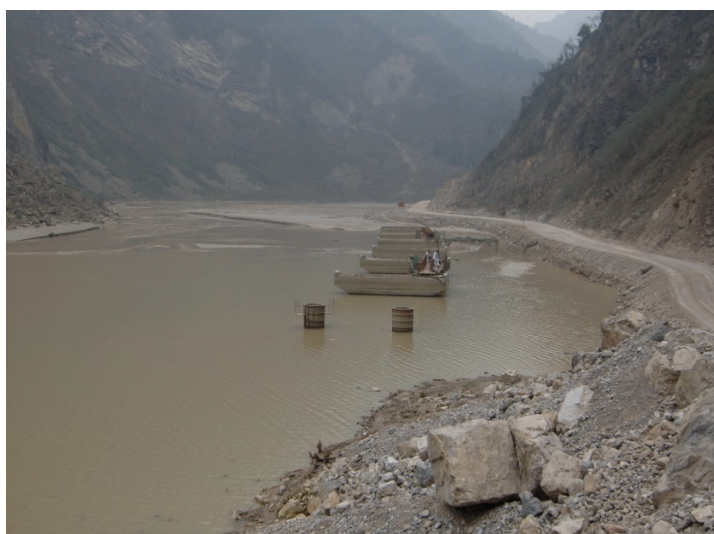
Figure 6. Dammed lakes preventing highway reconstruction at Mianyuan River.
