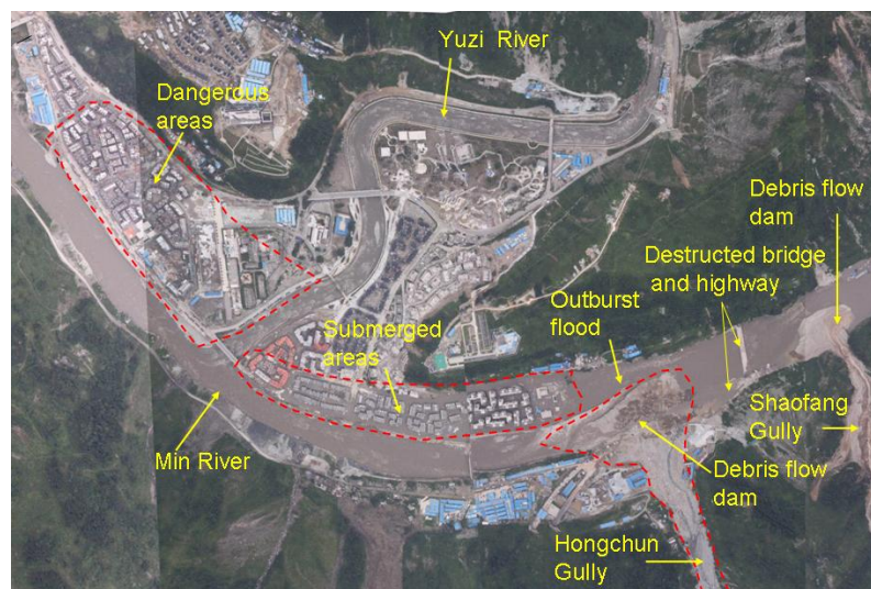
Figure 11. Yinxiu town threatened by 8.14 debris flows and outburst flood of dammed lakes.
