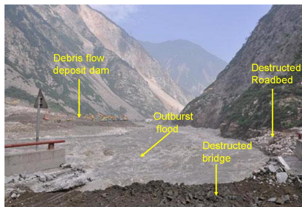
Figure 7. Outburst flood of dammed lake induced by Gaojia Gully destructed Dujiangyan-Wenchuan High-way at the outlet of Luoquanwan Gully.
