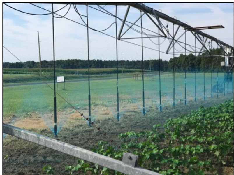
Figure 7. Injection of blue spray indicator being emitted through the LEPA drops nozzles.
