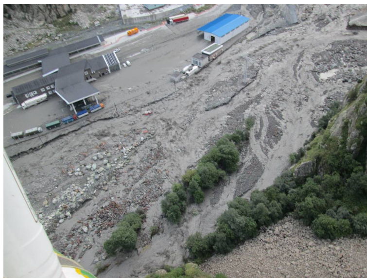
Figure 12. Damaged customs checkpoint building.
