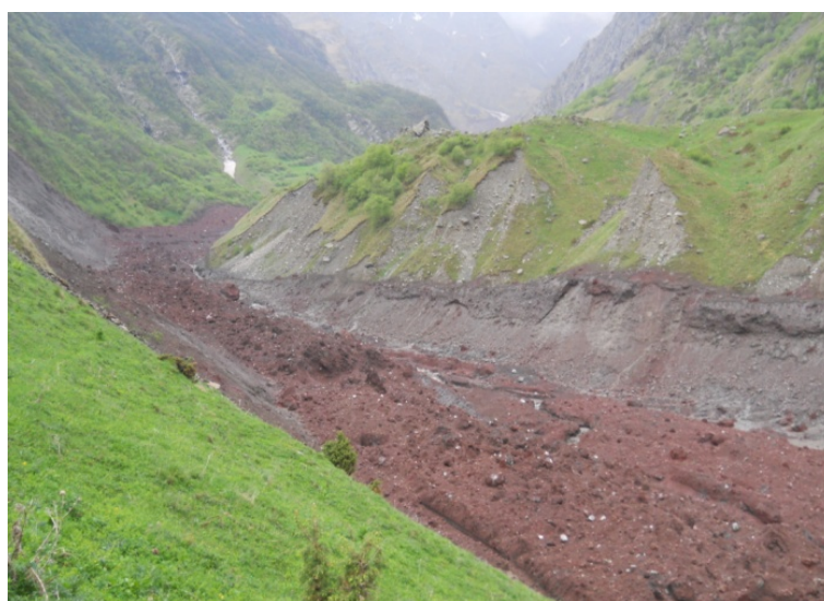
Figure 8. Accumulated debris material in Devdoraki Valley.
