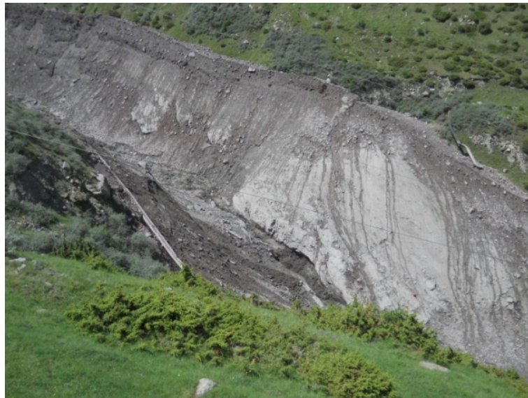
Figure 2. Destroyed gas pipeline.
