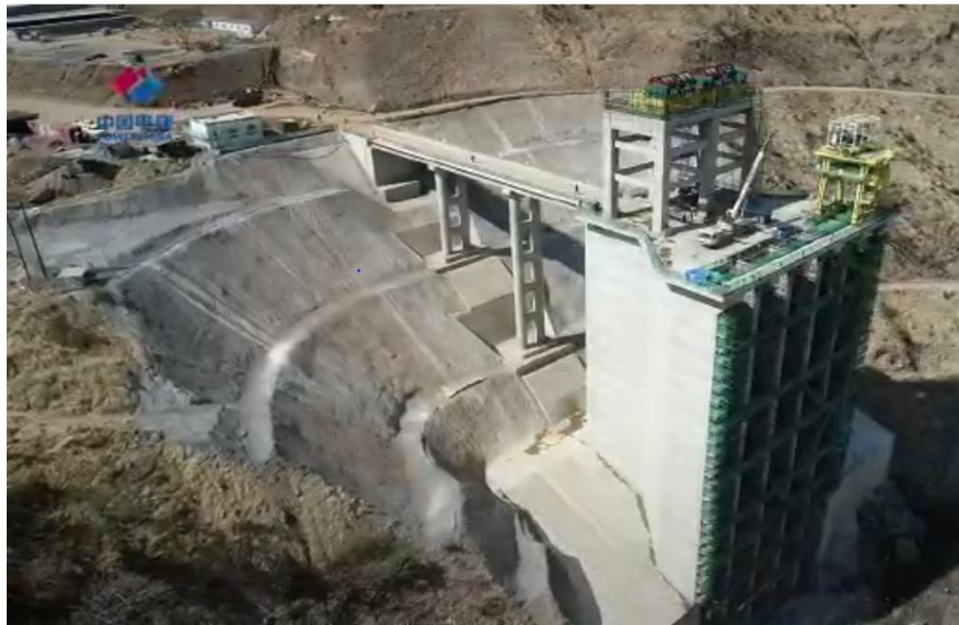
Photo 8. KGL Dam (intake view with water filled dam).
