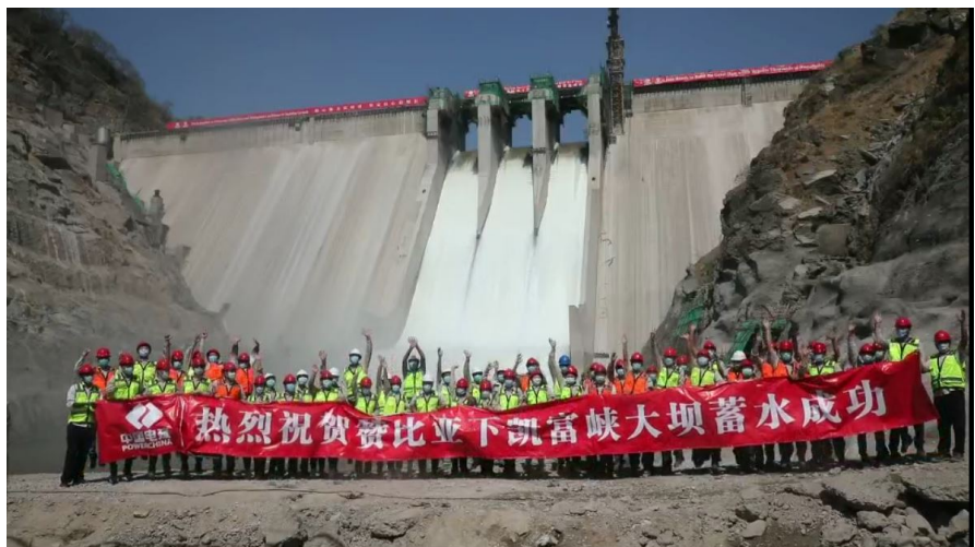
Photo 10. Completion of water filling of KGL Dam (downstream view).
