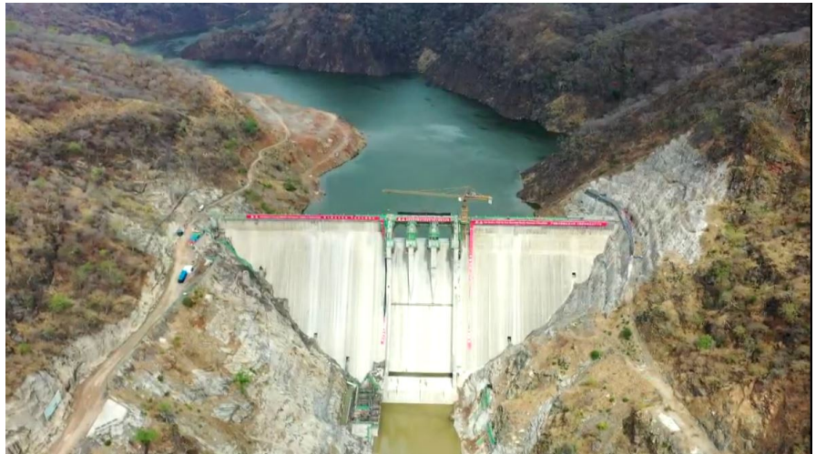
Photo 11. Completion of water filling of KGL Dam (plan view).
