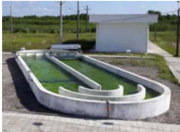
Figure 1. Cultivation of Scenedesmus sp. in raceways at UFRN.
