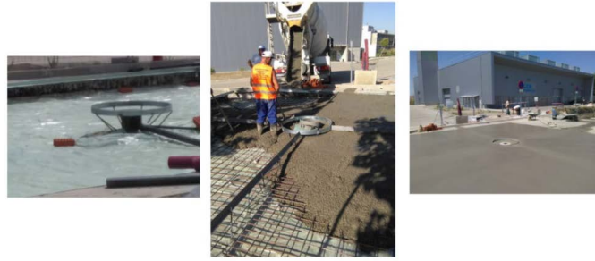
Figure 19. Concrete Slab construction images.
