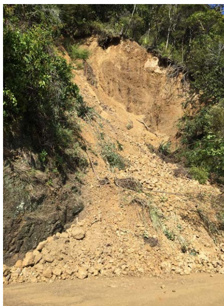
Figure 6. Over slip site 4.
