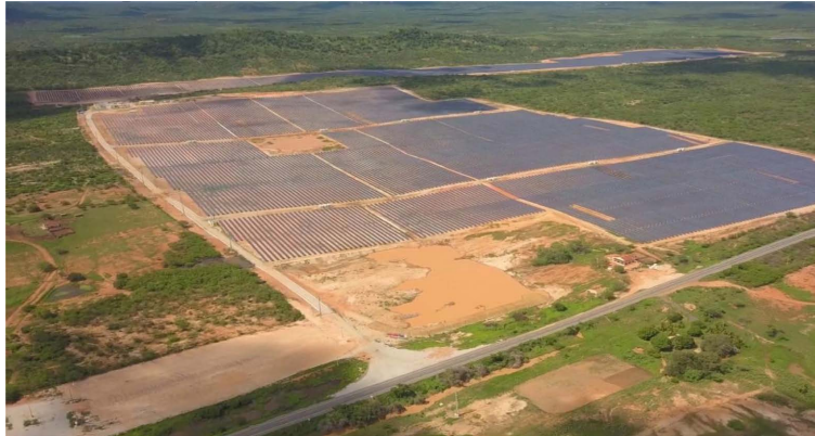
Figure 6. Aerial view of the Angico and Malta photovoltaic complex, Paraiba, Brazil.
