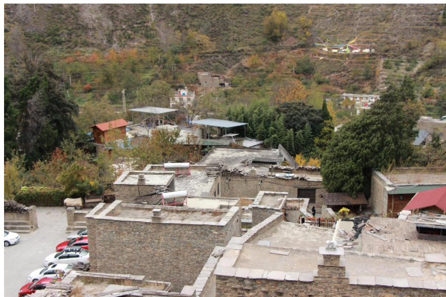
Figure 4. Taoping qiang village parking park (Photo by the author).
