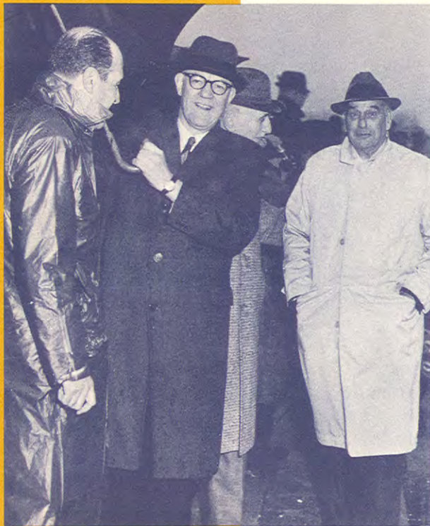
Rain notwithstanding, the first steel units for Unisphere's pedestal were erected in the presence of (left to right) Baron de Gunzburg, Eiffel Tower Corporation; Roger Blough, U. S. Steel; René Eiffel and Robert Moses, New York World's Fair.
