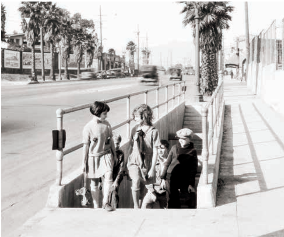
Micheltorena School Tunnel under Sunset (1927)
