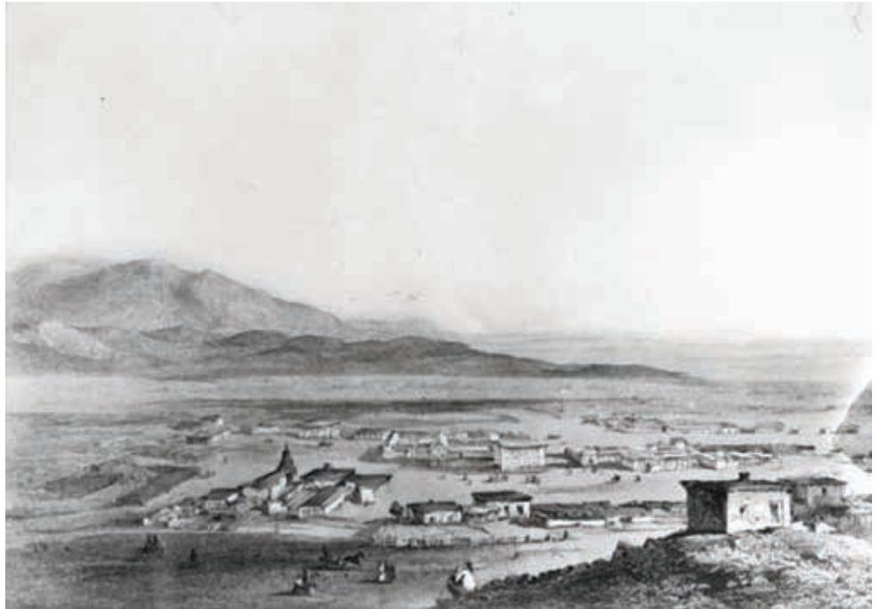
Eaton's Birthplace: Fort Moore Hill - The small house on the lower right of the screen is probably the adobe house where Fred was born in 1855. Drawing is of Los Angeles Plaza done in 1853 by Charles Koppel, looking east from Fort Moore Hill to the west, 1853.
