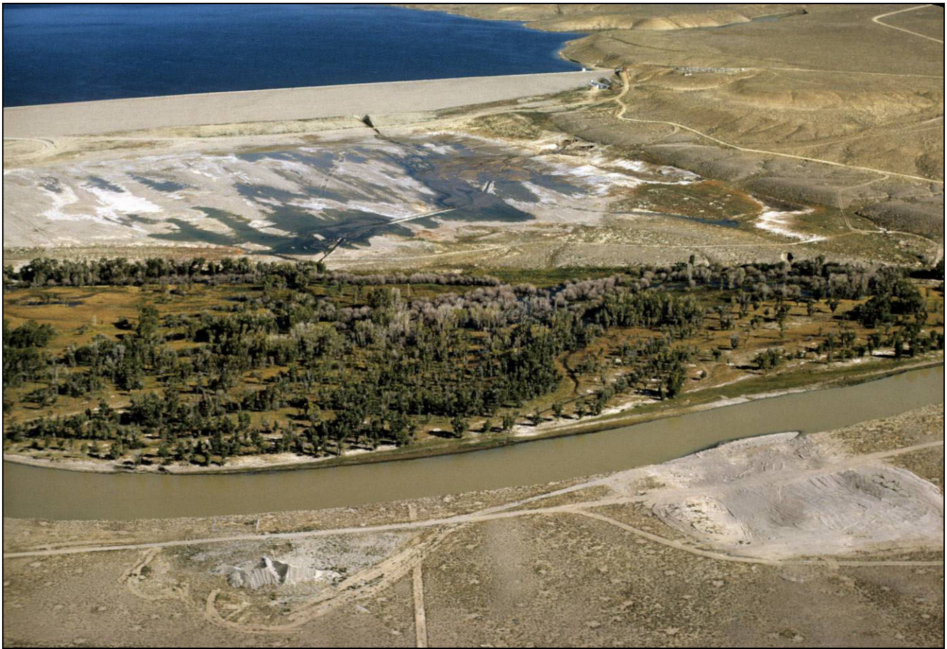
Figure 5. Fontenelle seepage downstream in 1965
