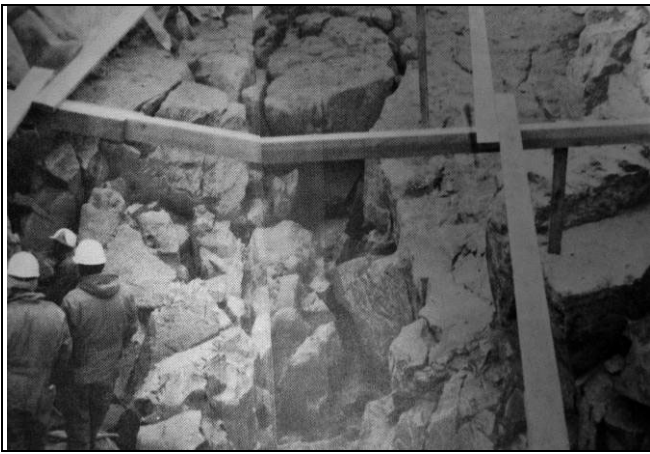
Figure 10A. Ririe construction photograph showing foundation in fault zone.
