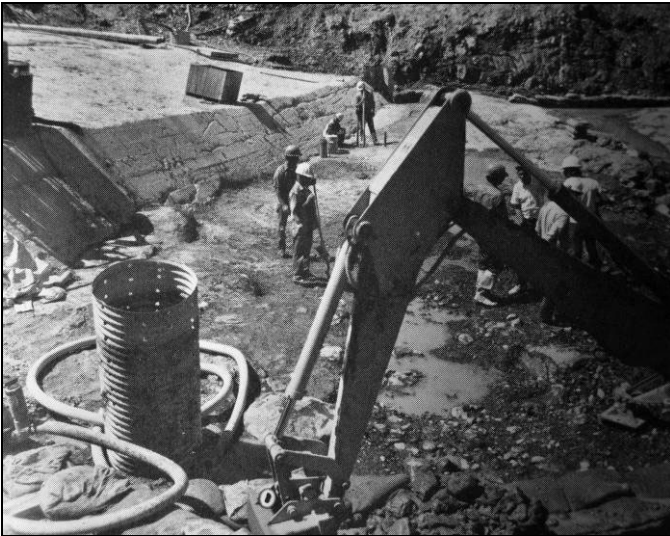
Figure 14A. Construction photo from Ririe showing dental concrete and foundation cleanup.
