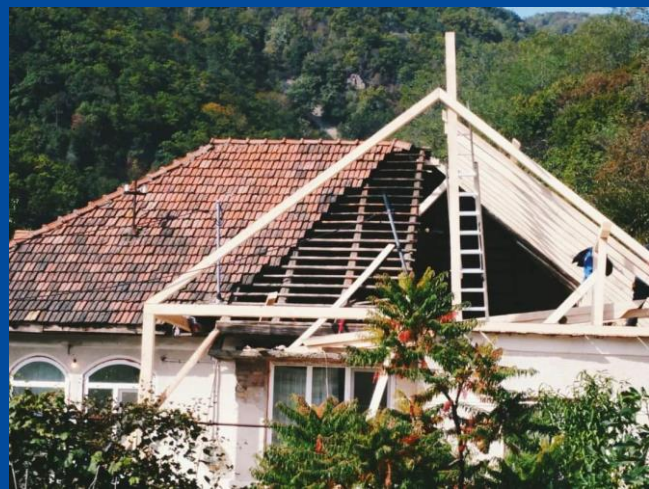
House being renovated in Bumbesti Jiu
