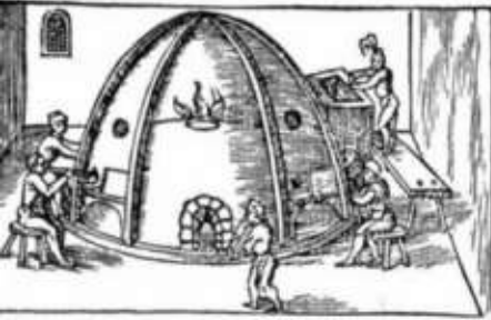
▲ Engraving of a Venetian glass furnace. From De la Pirotechnica by Vannoccio Biringuccio, 1540. The ingredients are being heated until molten and then blown into shapes.
