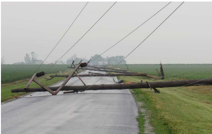
Since building the previous line 60 years ago, it had become outdated and Prairie Power could not replicate the original design.
