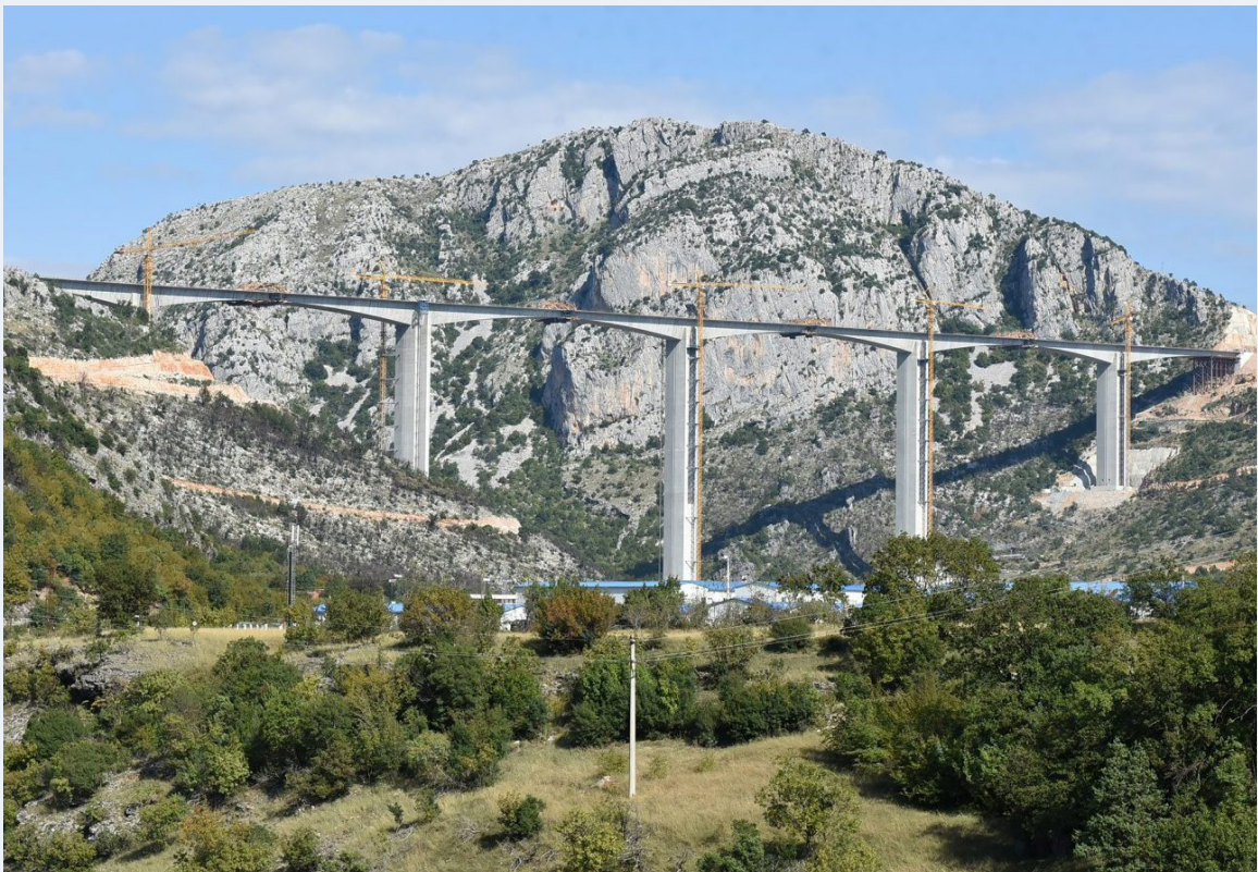
Komarnica bridge on the highway from Bar to Boljare in Montenegro.
