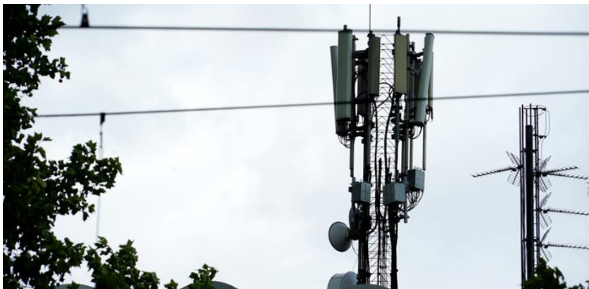
Telecoms infrastructure procured from Huawei by BH Telekom
