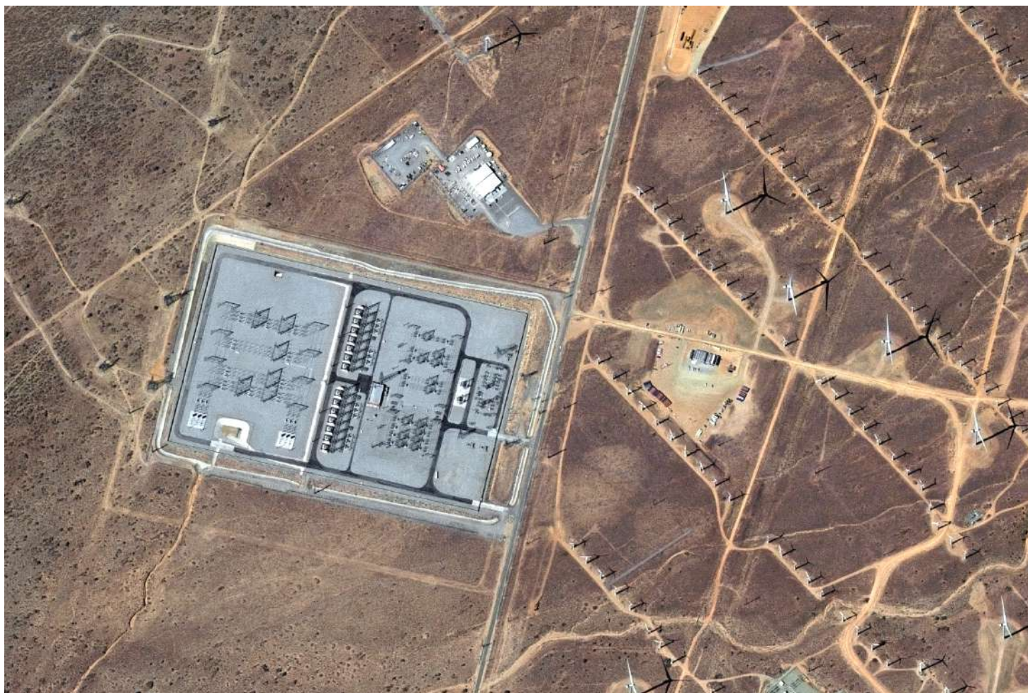
Figure 1: GEOSAT Image, Tehachapi Pass Wind Farm, Mojave, CA, US.
