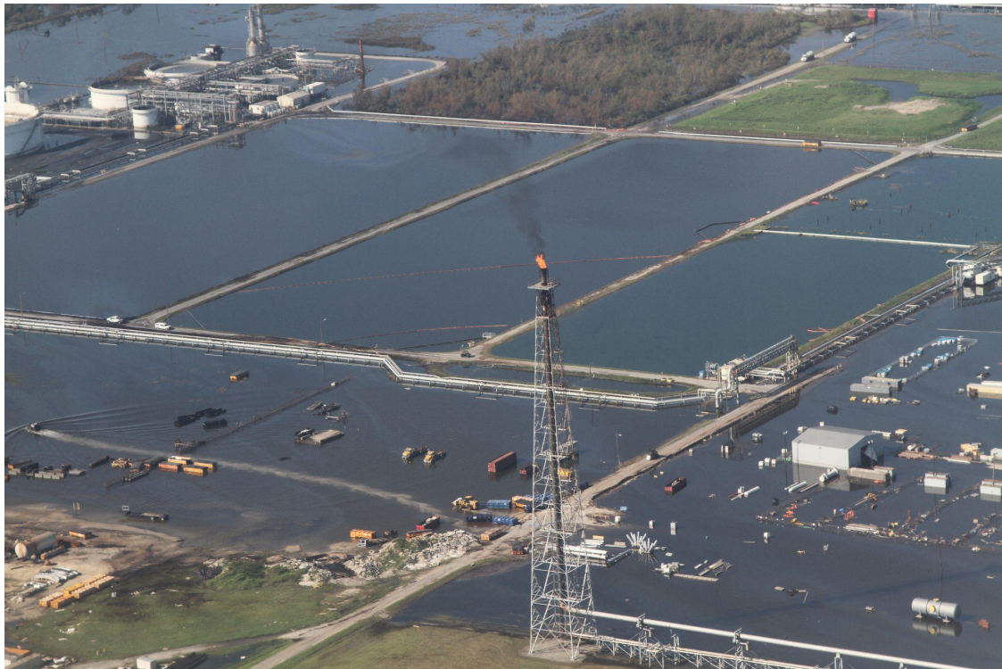
Figure 4. Phillips 66 Alliance Oil Refinery, 04 Sept 2021. The refinery is flooded and burns flares that smell of rotten eggs and are visible for many miles. Oil and chemicals pervade the flood waters - note the sheen in the upper left corner and the absorbent booms in the center pond. Photo: Healthy Gulf, % SouthWings.
