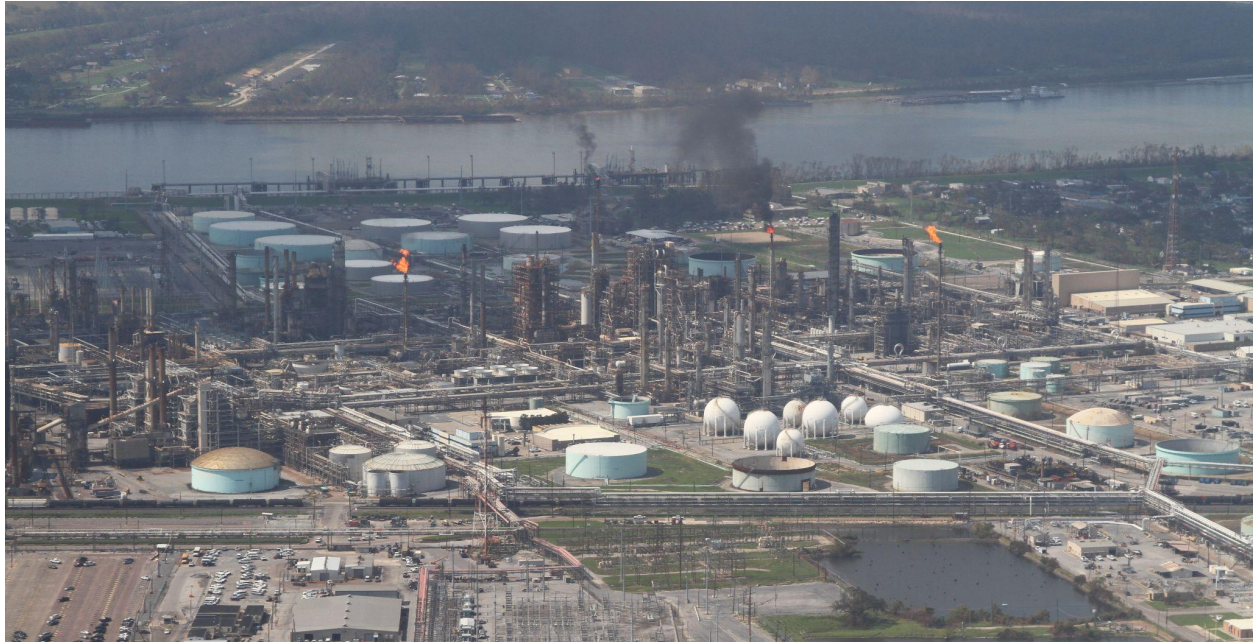
Figure 5. Norco Shell Oil Refinery, 04 Sept. 2021, burning at least four flares that smell of rotten eggs and send billowing black smoke into the air. Visibility is low due to the billowing smoke. Flares from this and other shuttered refineries and petrochemical plants were burning for weeks on end after the storm. Photo: Healthy Gulf, % SouthWings.
