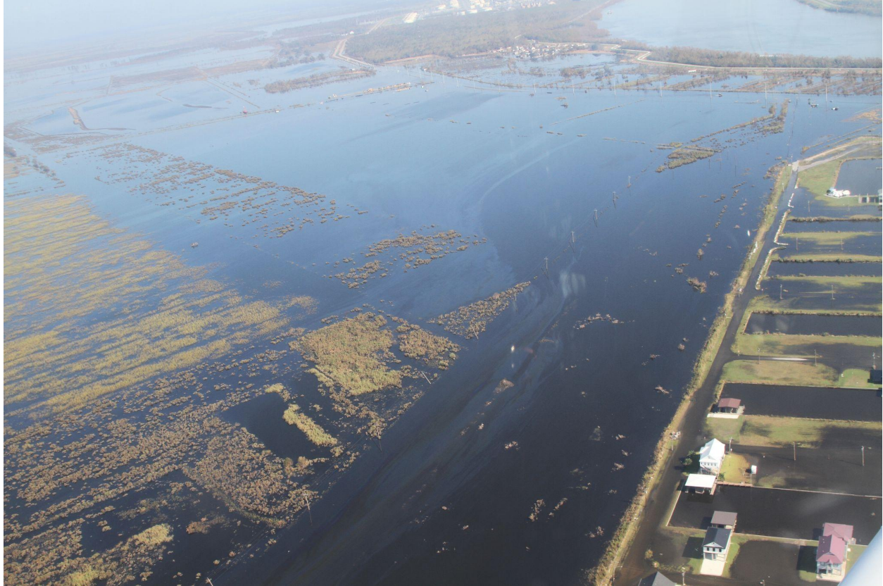
Figure 13. Fields between Ironton and Myrtle Grove Marina flooded with rainbow sheen streaks across the field. Highway 23 is underwater until just upstream of Ironton. The Phillips 66 Alliance Refinery is upstream, in the upper middle of the image. 04 Sept 2021, Photo: Healthy Gulf % SouthWings.
