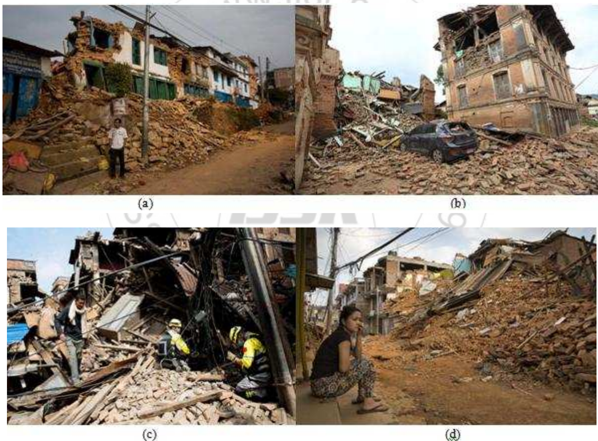
Figure 2: (a,b,c,d): The breadth of devastation in Nepal (25 April 2015 Earthquake)
