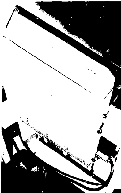
FIG. 9. Isolation transformers ("birdhouses").
