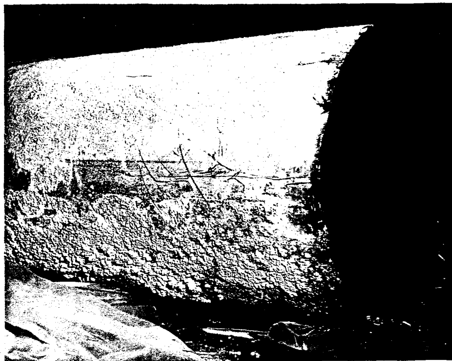
Fig. 4. The outside of the delay line pipe, cut near the surge tank, as found after excavation with the typical covering of rust-colored, nodular deposits.
