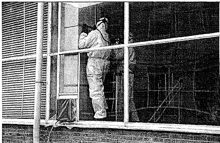
Photo 2 : Dismantling of ventilation pipes
