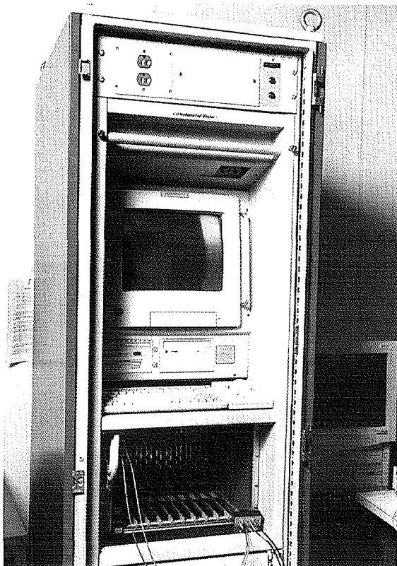
Figure 24 VIFB: CANDU Spent Fuel Bundle Counter electronics.
