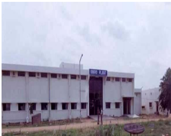
Fig. 1 View of SWRO Plant building and membrane modules
