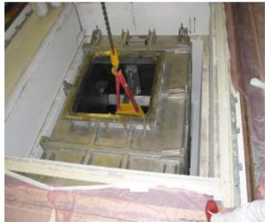
Figure 15. Stainless Steel Box(left) and Setting the Box into the Cell
