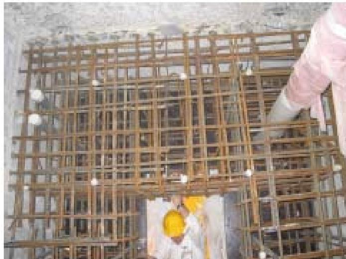
Figure 16. Strengthening of the Cell Bases for Seismic Withstanding Purposes(reinforced concrete).
