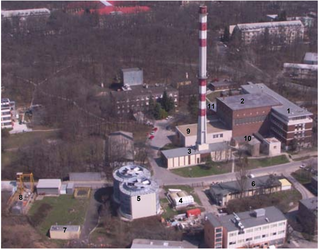
FIG. 1: Aerial view of the BRR site. 1) Reactor building with the control room being on the 2nd floor. 2) Reactor hall. 3) Engine room with air filters of the air ventilation system. 4) Secondary pump room. 5) Cooling towers. 6) Auxiliary building accommodating the diesel generators and compressed air system. 7) Building of the liquid waste storage facilities (under the foreground area two storage tanks are accommodated). 8) AFR-pool (with solid waste storage wells in the foreground area). 9) Cold neutron source (CNS) measuring hall. 10) Cryo-system of CNS. 11) Time-of-flight measuring hall.
