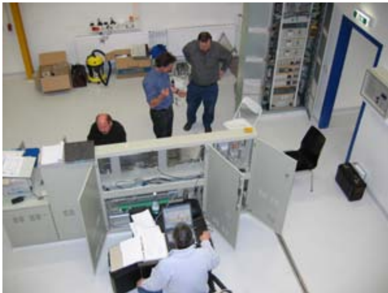
FIG. 5. Installation of I&C systems.
