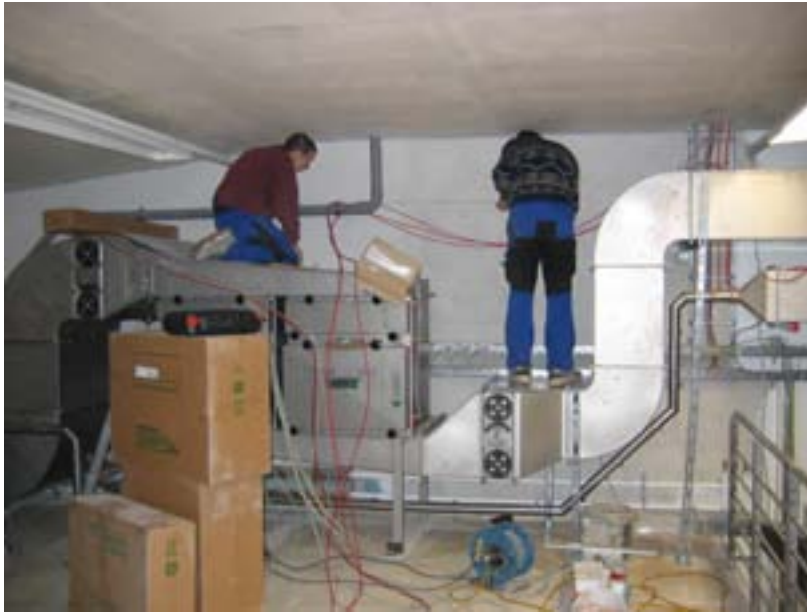
FIG. 4. Filter system of room ventilation.
