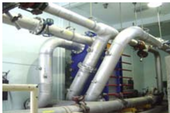
FIG. 4. Plate-type heat exchanger with modified piping arrangements.
