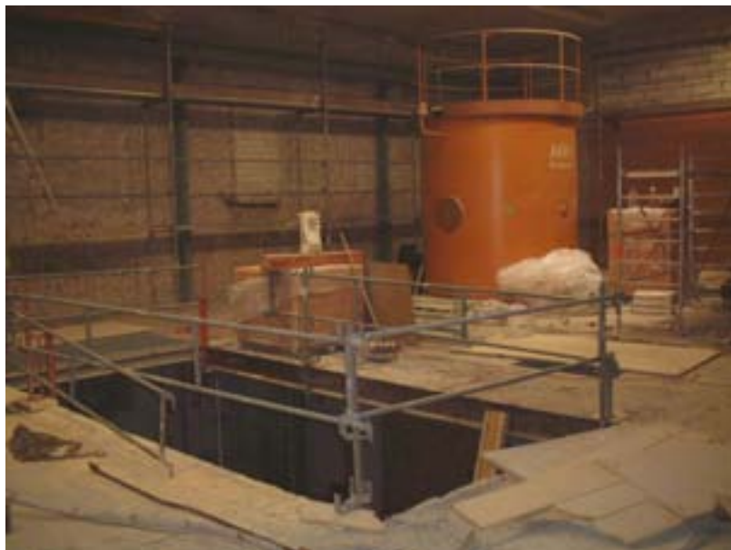
FIG. 3. Construction work in the reactor hall.
