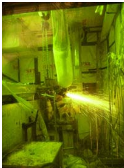
Figure 14: Remote grinding operations in shielded containment
