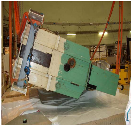
Figure 10: Canning Station Shell during Crane Lift
