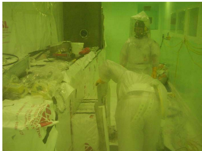
Figure 22: A two-piece Air Fed Suit being worn during decommissioning activities
