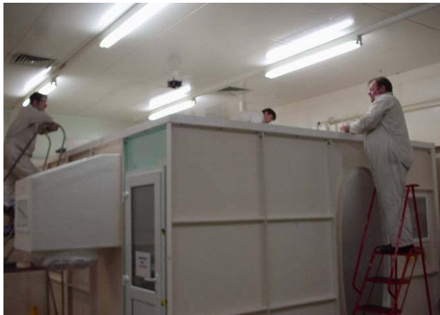
Figure 5: Glove-box prepared for decommissioning
