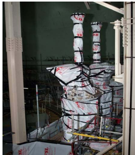
Figure 9: Charge Machines on Canning Station ready for removal
