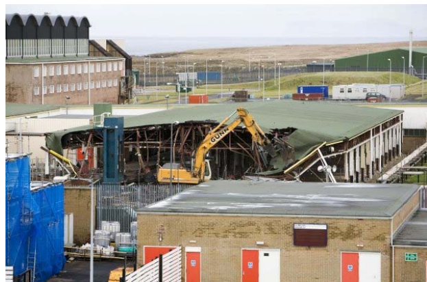
Figure 27: Demolition of fuel fabrication plant
