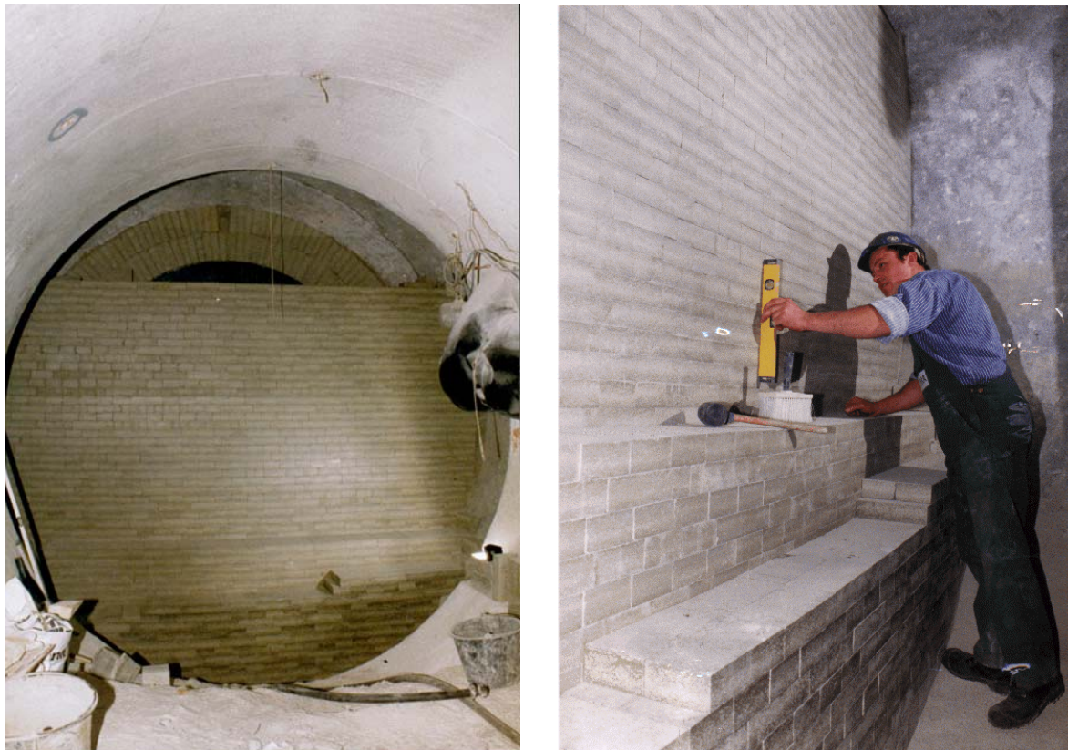
Figure 1: Emplacement of bentonite sealing elements in rock salt.
