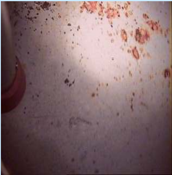
(oxide particles deposit on the pool bottom next to beam port No #3 )
