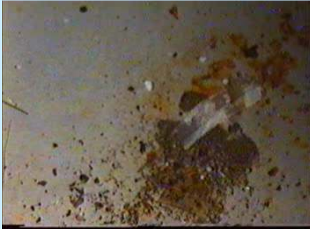
On the pool bottom before cleaning (2001)
