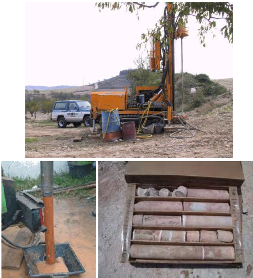
Figure 4. Images of diamond core drilling (top), core extraction (bottom left) and core tray (bottom right).
