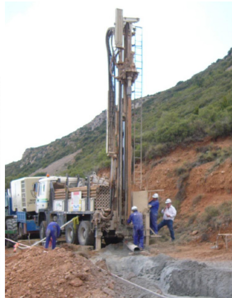
Figure 3. Basic operation scheme (left) and image (right) of percussion rotary drilling.
