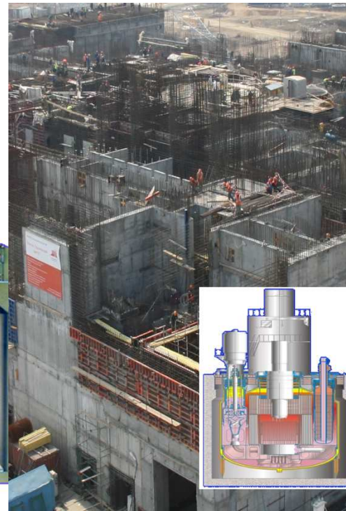
BN-800 Construction - by 2014
