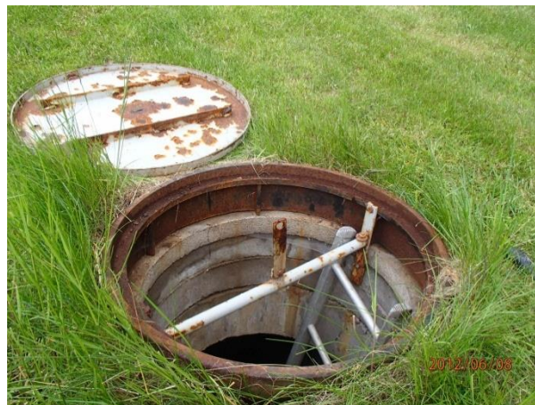
Figure 3. Inspection well with manhole cover and ladder.
